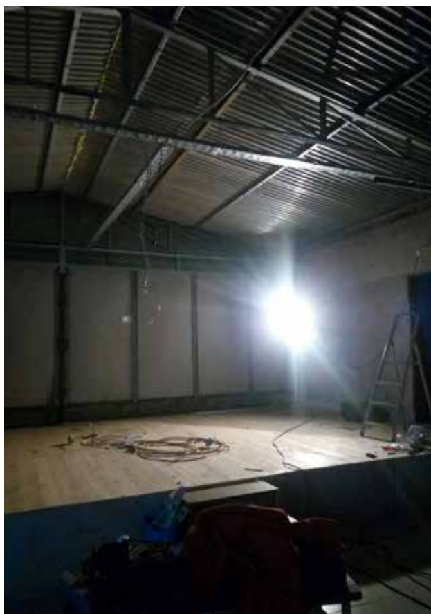
As obras do palco
